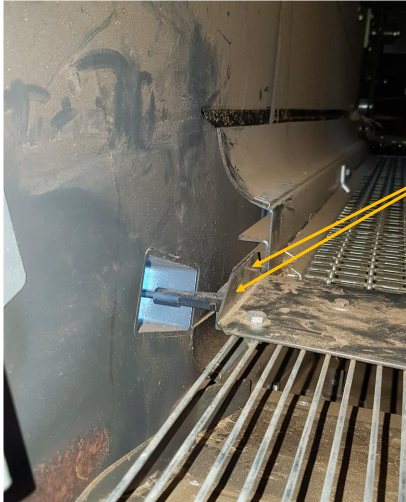
Before installing shroud
